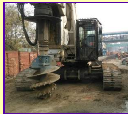
Foundation, Piling and Geotechnical
