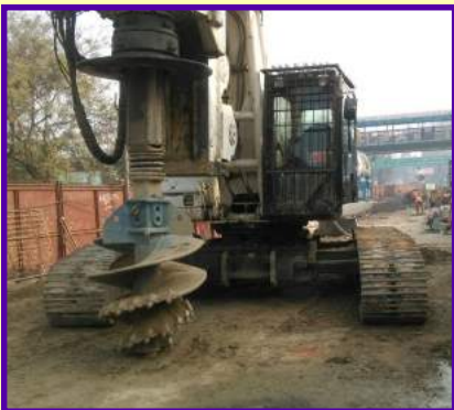
Foundation, Piling and Geotechnical
